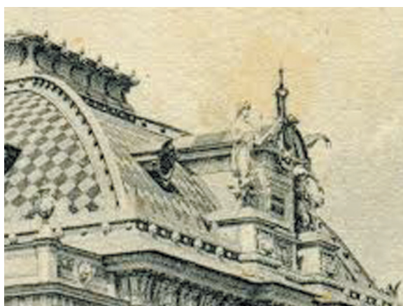
A part of the Noble Assembly’s building.
