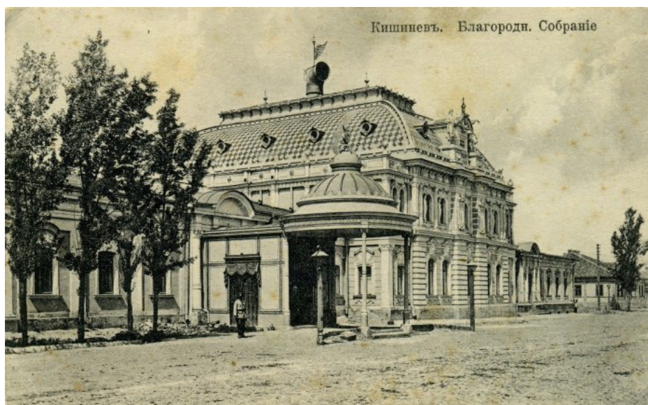
The bulding of Noble Assembly in Chișinău. Arhitect H. Lonsky.
